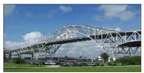
Corpus Christi Harbor Bridge, a Through Truss and Deck Truss Structure, is 1782 feet in Length
