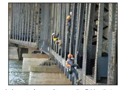
HDR Inspectors used Rope Access Techniques to Access Areas on the Bridge that would not be Accessible using Traditional Methods
