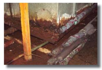
Damage on the Exchanger due to cooling water leak
