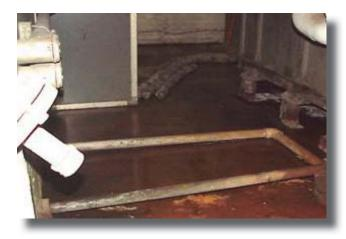
Flooding in the mechanical room from cooling water leak
