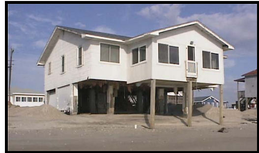
Figure 17-2. This coastal building suffered extensive damage to the enclosed lower area.
