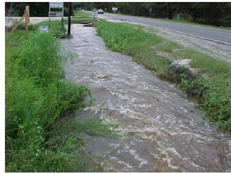
Figure 28-4. Good drainage maintenance allowed this ditch to do its job during Tropical Storm Isidore in 2002.
