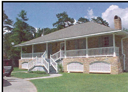
Figure 28-7. Owners as funders: This is one of five structures in Denham Springs that were elevated in 1995. The owners paid approximately 52% of the cost, up to $40,000 each. They all escaped damage
