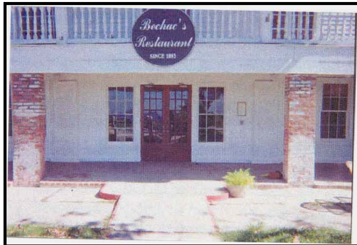
Figure 12-1. This floodproofed restaurant in Mandeville is an example of where human intervention is needed. Protecting this nonresidential building is dependent on installing a doorway barrier in time.
