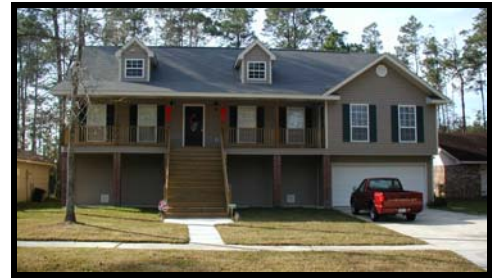
Figure 28-2. This Louisiana home was elevated with DHS/FEMA funds.
