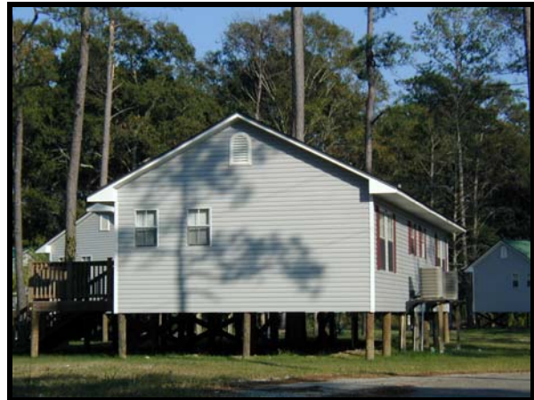
Figure 11-3. House elevated on piers (Slidell).
