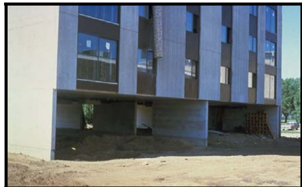
Figure 11-4. Elevation on parallel walls.
