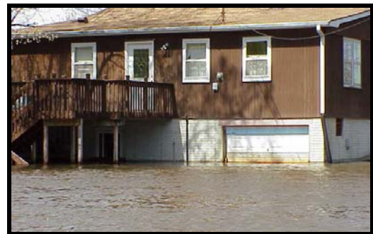
Figure 17-3 This house was properly elevated. Some time after the permit was issued, the owner improved the lower area and subsequently suffered flood damage. This shows the benefit of requiring lower areas to stay open.
