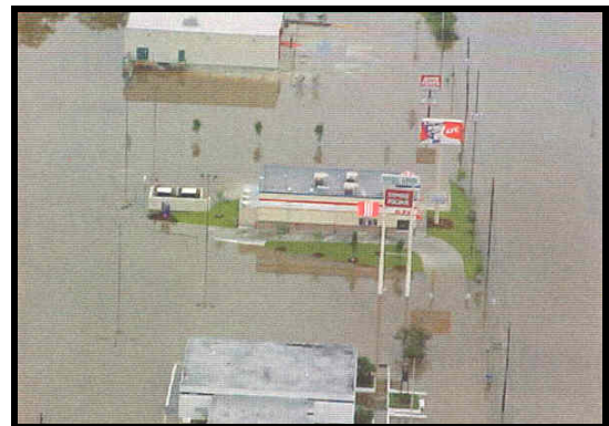
Figure 11-2. This KFC restaurant in East Baton Rouge Parish was built on fill according to the parish's floodplain management ordinance. There was no water in the building during Tropical Storm Allison in 2002.
