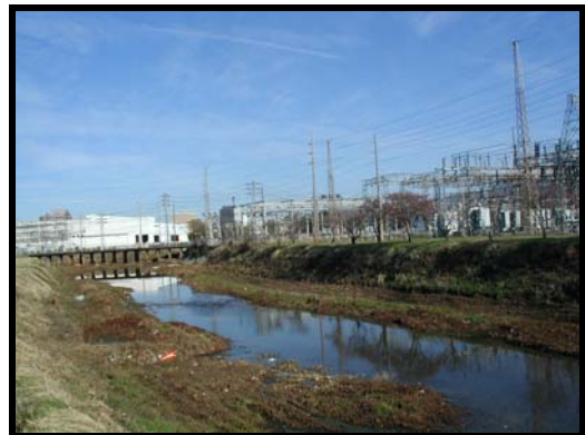
Figure 17-5. Example of a critical facility in the floodplain.
