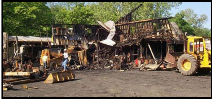
Figure 2-3. A propane tank floated into this building, exploded, and destroyed it.
