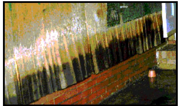
Figure 2-11. Prolonged exposure to water and “wicking” can destroy wood and gypsum walls.
