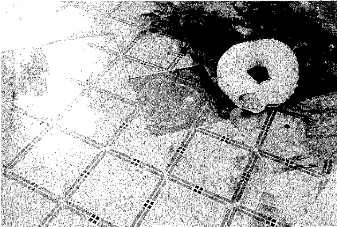
Photo 3 View of multiple layers of flooring.
