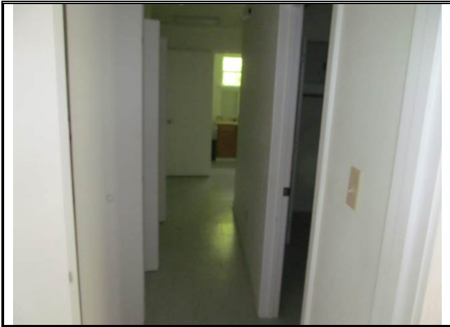
Photograph No. 013: Hallway overall
