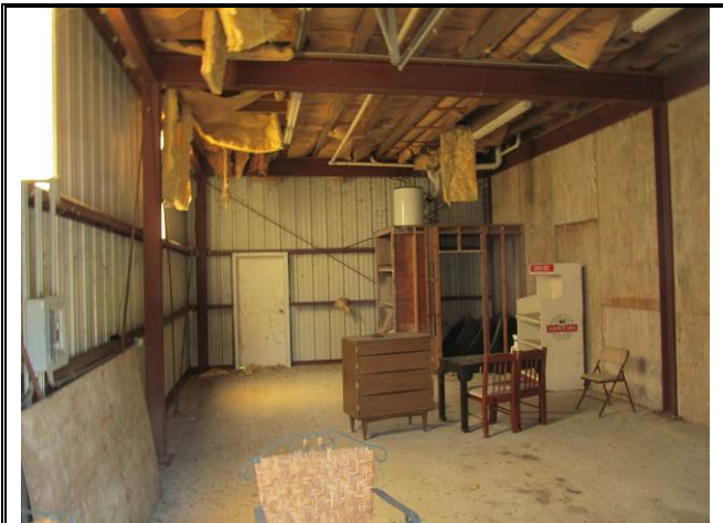
Photograph No. 002: Garage Overall
