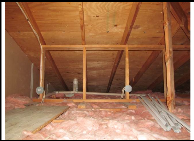
Photograph No. 019: Attic Overall
