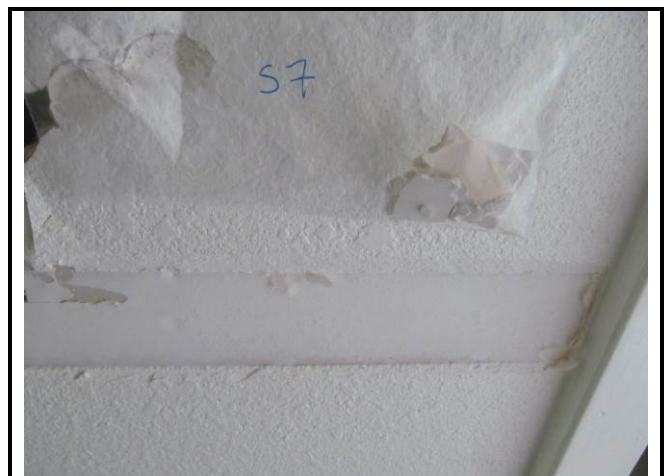
Photograph No. 018: Sample 7 – Drywall joint compound
