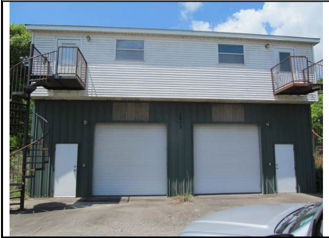
Photograph No. 001: Overall exterior
