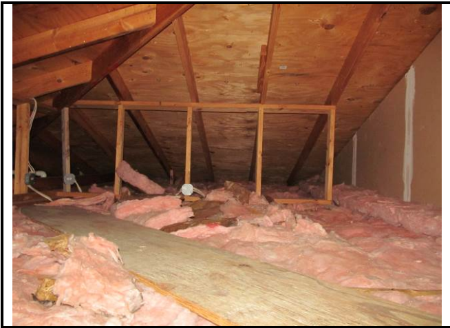
Photograph No. 020: Attic Overall
