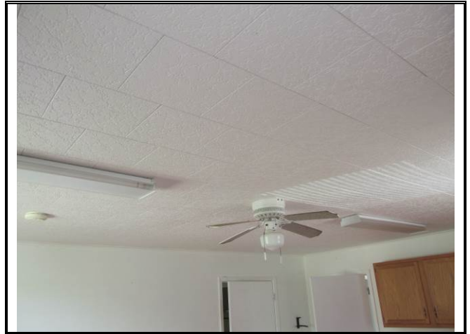
Photograph No. 016: Drop ceiling tile overall
