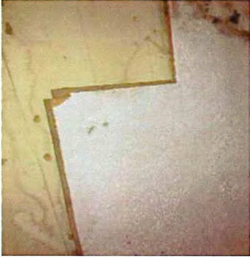
Photograph No. 6 View of popcorn ceiling texture over white ceiling tile in the Kitchen.
