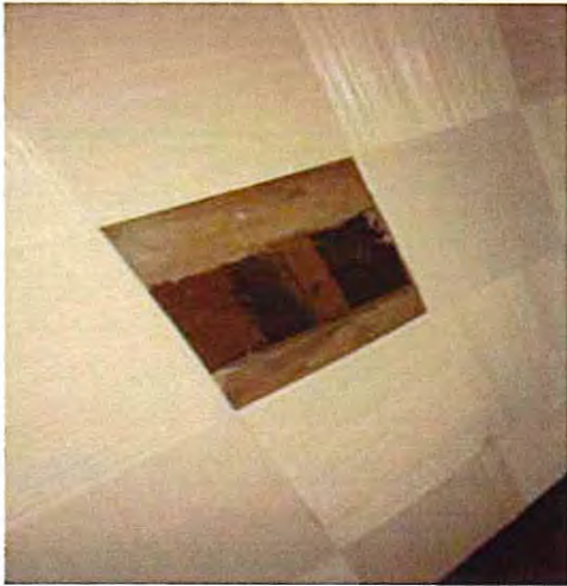
Photograph No. 5 View of brown vapor barrier above living room ceiling.
