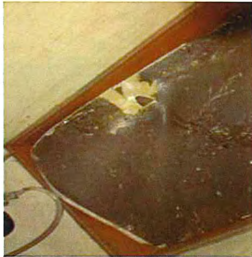
Photograph No. 7 View of gray speckled sheet flooring in Bath #1 and Bath #2 on the first floor.
