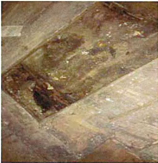
Photograph No. 9 View of brown vapor barrier below wood flooring on first floor.
