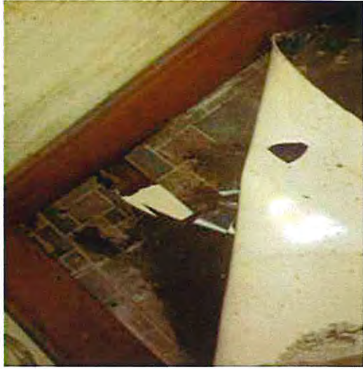
Photograph No. 6 View of popcorn ceiling texture over white ceiling tile in the Kitchen.
