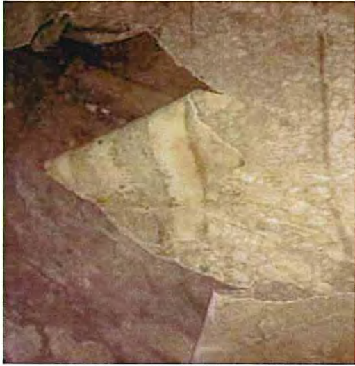
Photograph No. 10 View of beige sheet flooring in Dining Room on first floor.
