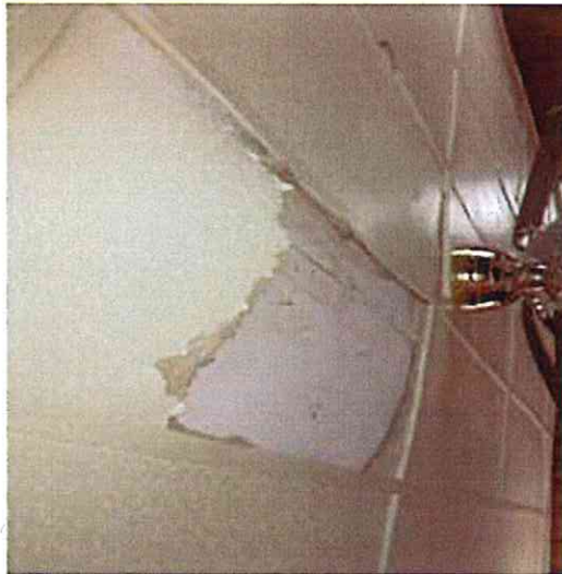
Photograph No. 11 View of 2' x 4' pinhole ceiling tile on second floor.
