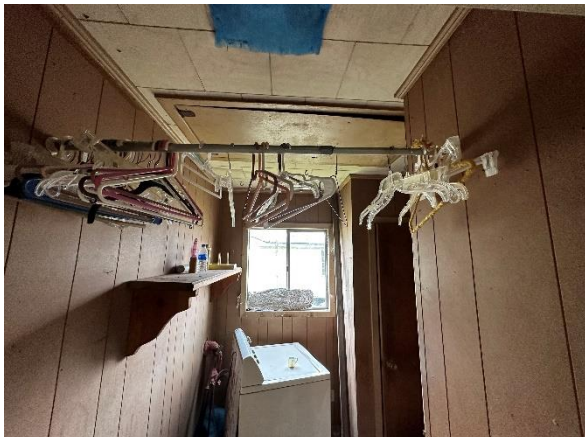
Photo #9: General view of the laundry room area
