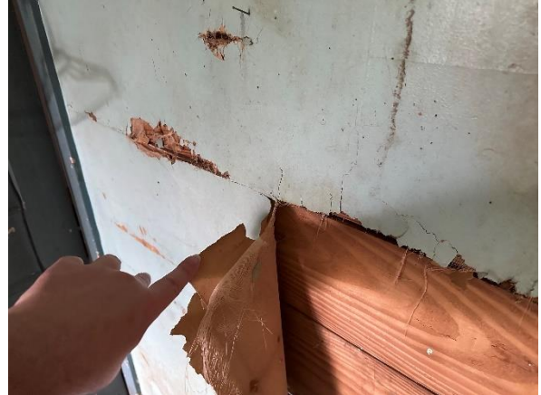
Photo #8: View of HA-8 – Woven wall covering on wood walls
