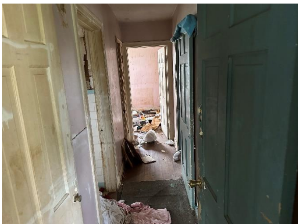
Photo #11: General view of the hallway
