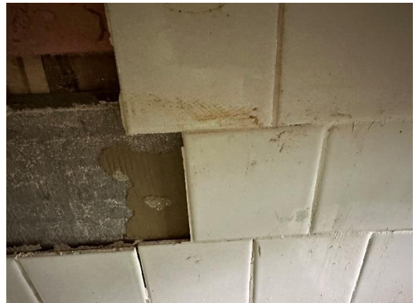
Photo #4: View of HA-4 – 4x4 White bathroom tile with associated thin set/grout
