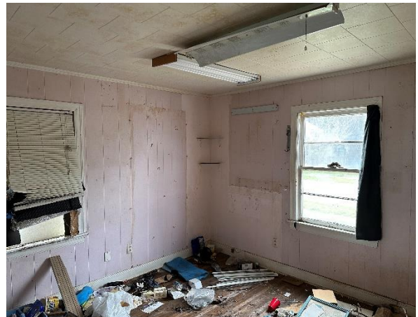
Photo #12: General view of bedroom #1
