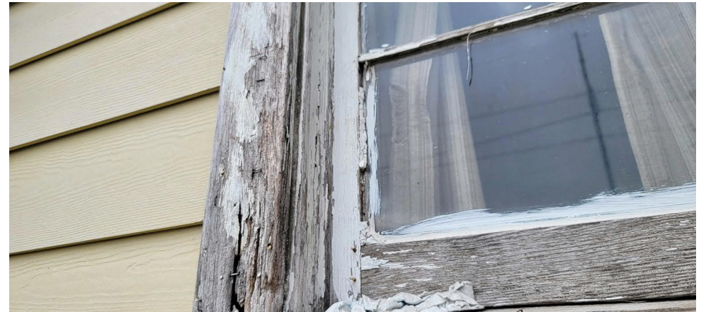
Photograph No. 16 HA-18: White Window Caulking
