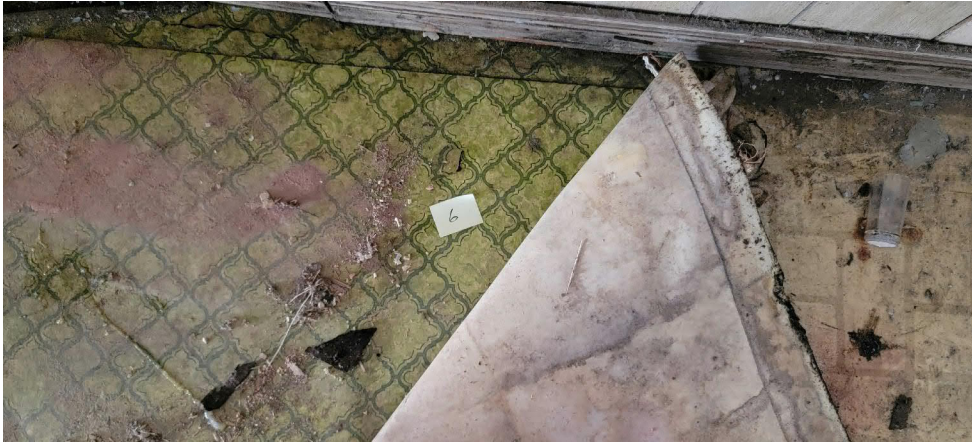
Photograph No. 5 HA-06: Green Pattern Vinyl Sheet Flooring
