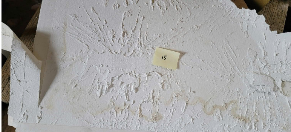
Photograph No. 13 HA-15: White Wallboard Ceiling with Spackle Texture
