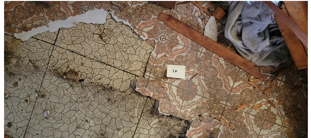
Photograph No. 8 HA-10: Brown/White Pattern Vinyl Sheet Flooring
