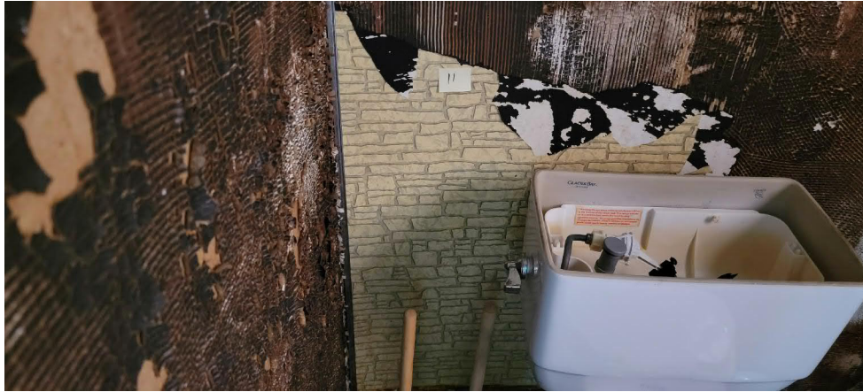
Photograph No. 9 HA-11: White Vinyl Wall Sheeting with Black Adhesive
