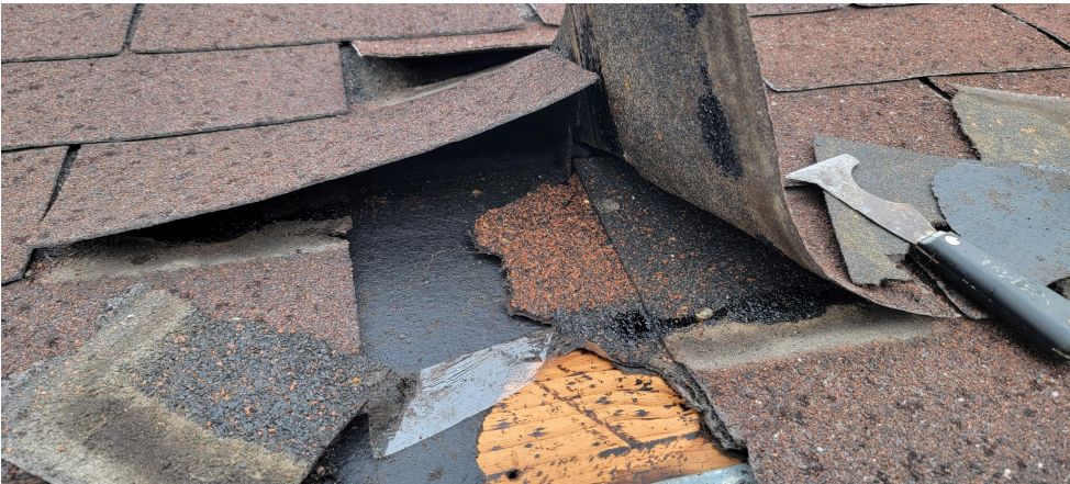
Photograph No. 15 HA-17: Red Roof Shingles with Black Tar Paper
