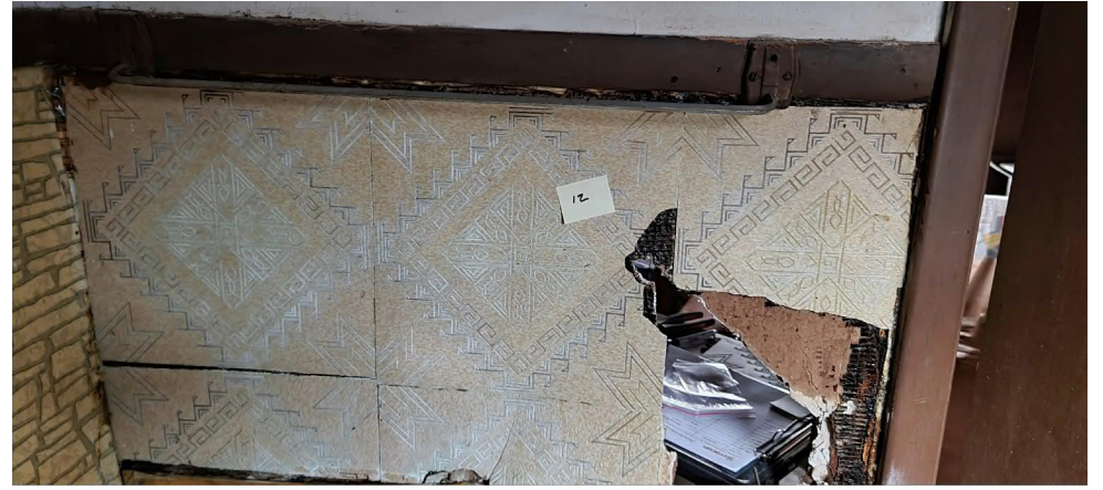
Photograph No. 10 HA-12: Beige Pattern Wall Sheeting with Black Adhesive
