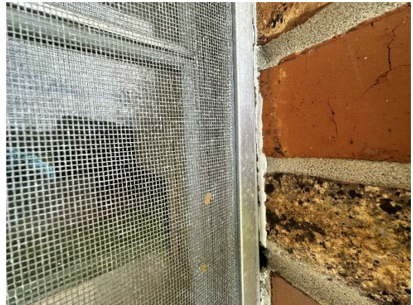
Photo #14: HA-14: White window caulk
