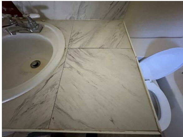
Photo #13: HA-13: 12"x12" White and grey floor tile with associated mastic (used on countertop)
