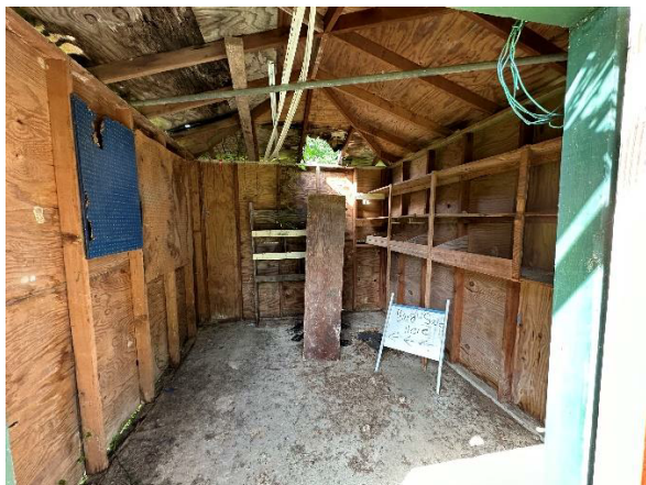
Photo #17: View of shed interior
