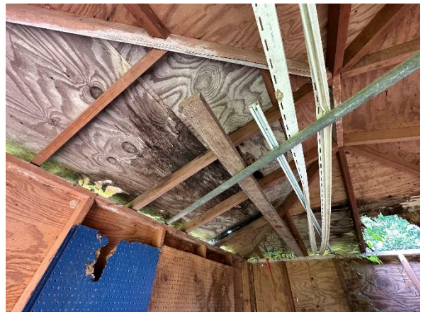
Photo #18: View of shed roof from the interior
