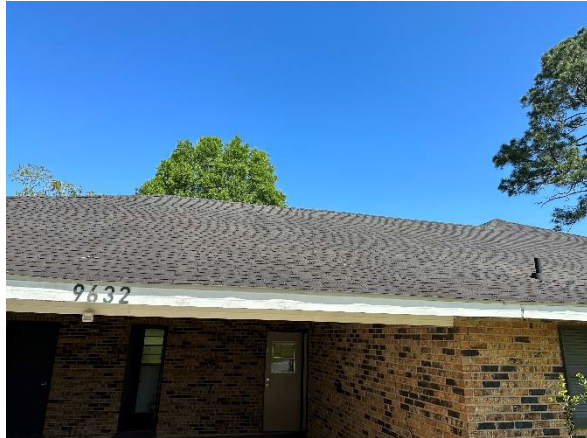
Photo #1: HA-1: Black roofing shingles (from House)
