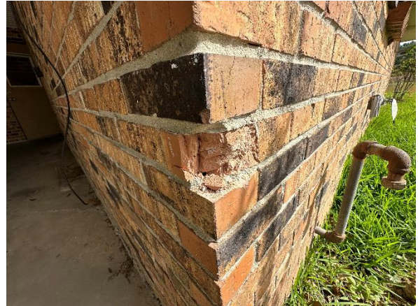
Photo #2: HA-2: Grey exterior brick mortar
