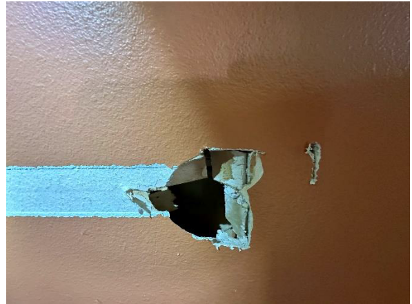
Photo #8: HA-8: Wallboard system with texture (could not separate texture)
