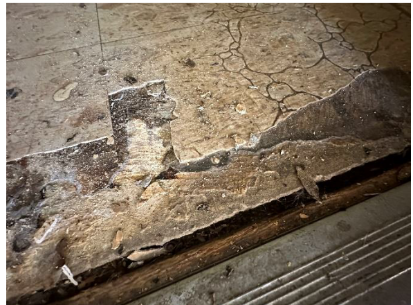
Photo #4: HA-4: Black floor tile with associated mastic (Under HA-3)
