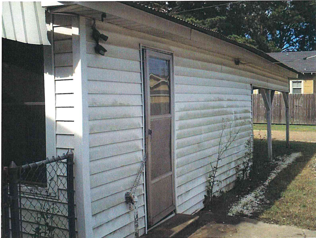
Photo 3 View of storage area of garage.
