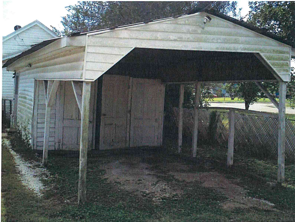
Photo 1 View of structure with attached car port.
