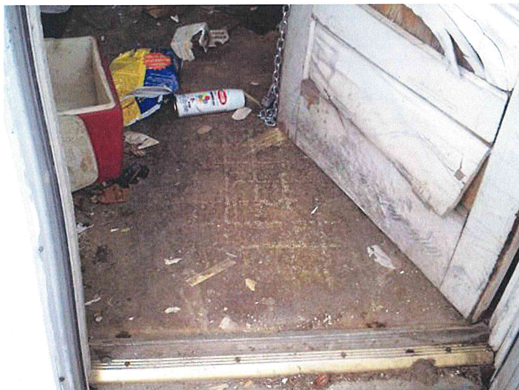
Photo 4 View of HA-2: ACM linoleum floor tile
