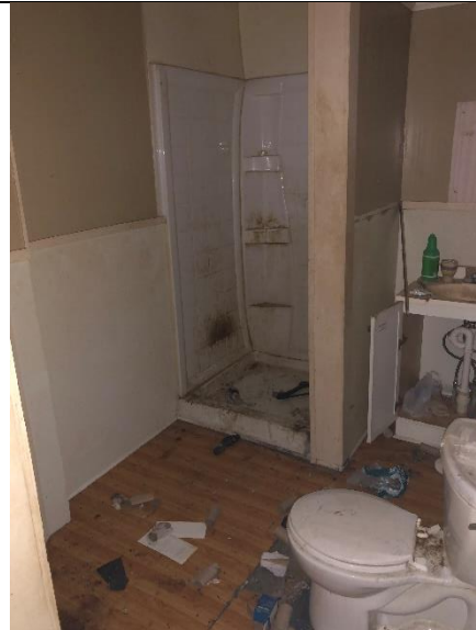
425 Sampson St – Master Bathroom
