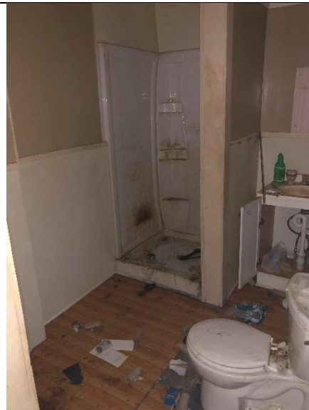
425 Sampson St – Master Bathroom
