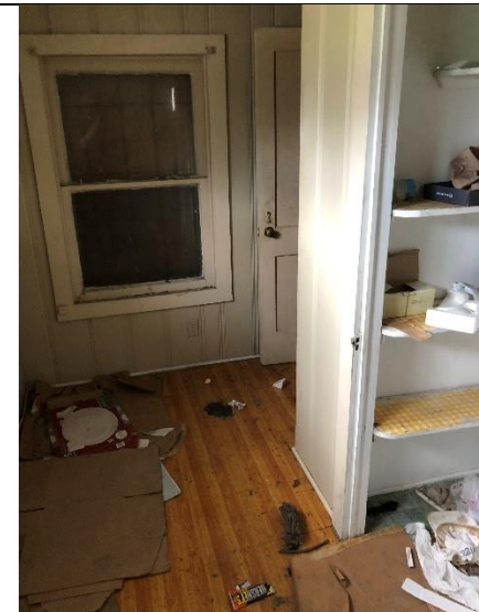
425 Sampson St - Addition
