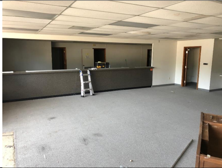
400 Mudd Ave - Lobby
