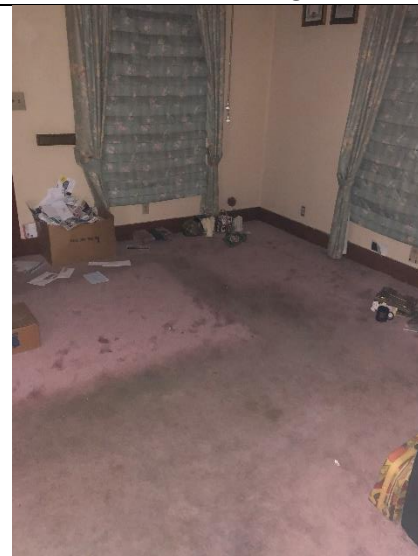
212 First St – Front Bedroom
