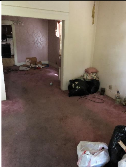
212 First St – Foyer
