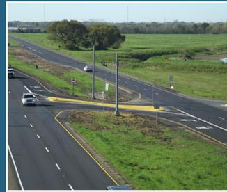
The J-turn concept is a reconfiguration of the traditional intersection that is used in different parts of the country to improve traffic flow. DOTD has begun using this concept at specific locations across Louisiana.
