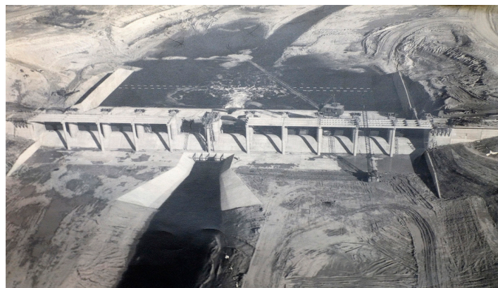
Toledo Bend Dam being constructed above.
