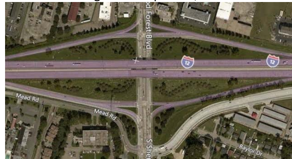
“DIAMOND INTERCHANGE” If the general north direction is to the right of the picture...
