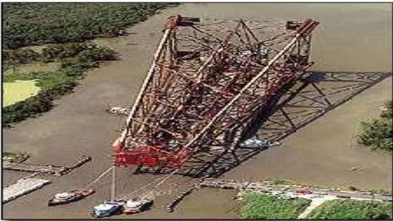
Oil rig built in Houma being moved down the Houma Navigation Canal to the Gulf of Mexico
