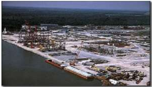
Gulf Island Fabricators' facilities in Houma
